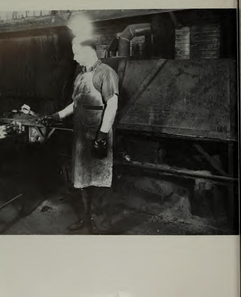
After any remaining babbitt is chipped off with a chisel, the bearing end of the rod is then dipped into a solution of hydrochloric acid. The acid acts as a cleaning agent. The acid vat is under the wooden cover shown at the right in the above picture. Then the bearing end of the rod is dipped into a molten tin or solder shown on the left in the above picture. This solder or tin acts as a flux or bond when the babbitt is cast against it.
